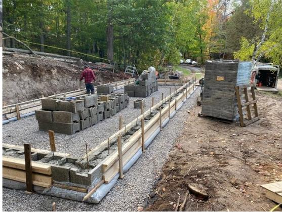
**NEXCEM BASEMENT WALLS** — A Nexem block is the only ICF that isn't made of foam or polystyrene (high carbon emissions). It is made here in Ontario from waste wood chips and some cement. But a portion of the carbon emissions are offset by the wood chips (trees sequester carbon) mixed in with the Nexem blocks. The cement protects the wood from decay while the wood adds insulation.
