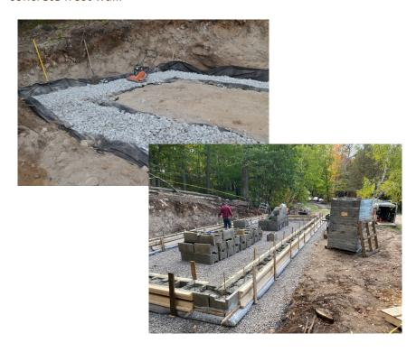
**NEXEM BASEMENT WALLS** — A Nexem block is the only ICF that isn't made of foam or polystyrene (high carbon emissions). It is made here in Ontario from waste wood chips and some cement. But a portion of the carbon emissions are offset by the wood chips (trees sequester carbon) mixed in with the Nexem blocks. The cement protects the wood from decay while the wood adds insulation.
