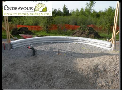
A poured slag-cement perimeter beam (right) uses sono tubes to displace concrete use. Next time, we'll lay a single tube horizontally. An earthbag foundation is used under the curved wall section.
