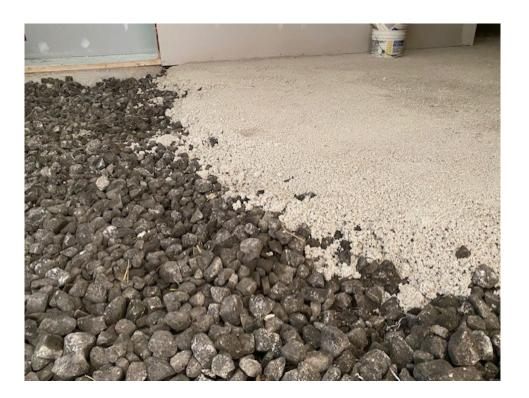
**GLAVEL AND PORAVER** — The basement floor of the Rotary Health Centre is insulated with two different types of recycled glass that otherwise might have ended up in the landfill. Glavel and Poraver are both made by heating and expanding glass into insulation suitable for below-grade applications.
