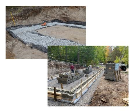
**NEXCEM BASEMENT WALLS** — A Nexem block is the only ICF that isn't made of foam or polystyrene (high carbon emissions). It is made here in Ontario from waste wood chips and some cement. But a portion of the carbon emissions are offset by the wood chips (trees sequester carbon) mixed in with the Nexem blocks. The cement protects the wood from decay while the wood adds insulation.
